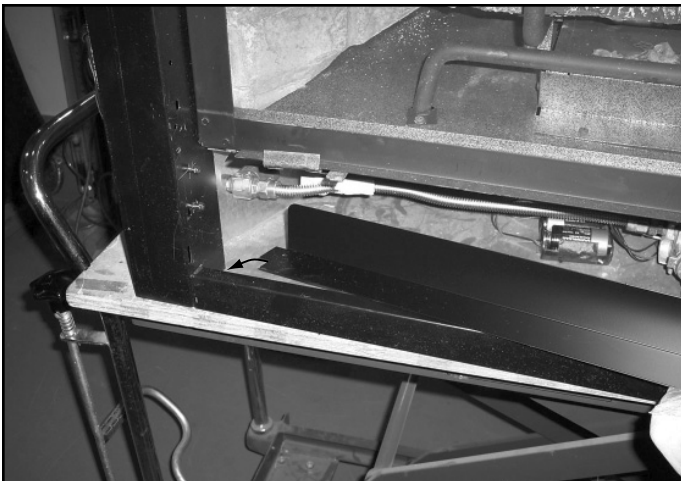
Figure 14.10 Installing Floor Cover
